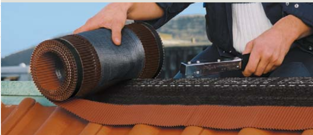
1. DELTA®-VENT ROLL am First antackern.
